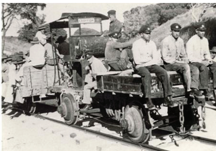
Above Top: Manual construction of the railway, including use of horse drawn scoops | Above Bottom: A working party being transported to the Oliver Hill gun Battery from the Barracks in 1937 by locomotive "Crayfish". Engineering personnel are on the locomotive; artillery personnel on the railway truck.
