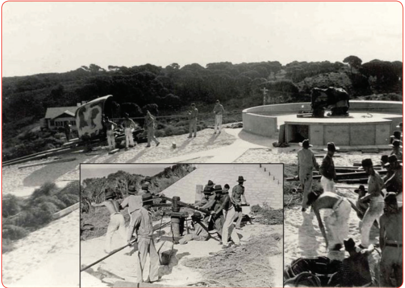
Bickley Point - Hauling the Bickley No 1 gun shield onto the gun position after it has been unloaded from the railway trolley. Personnel are using a timber sleigh on rollers that is being hauled up with a grab capstan (just in view on right - see inset).
