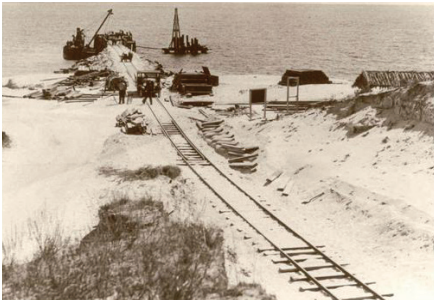
Early Stages of the Jetty upgrade, 1935.
