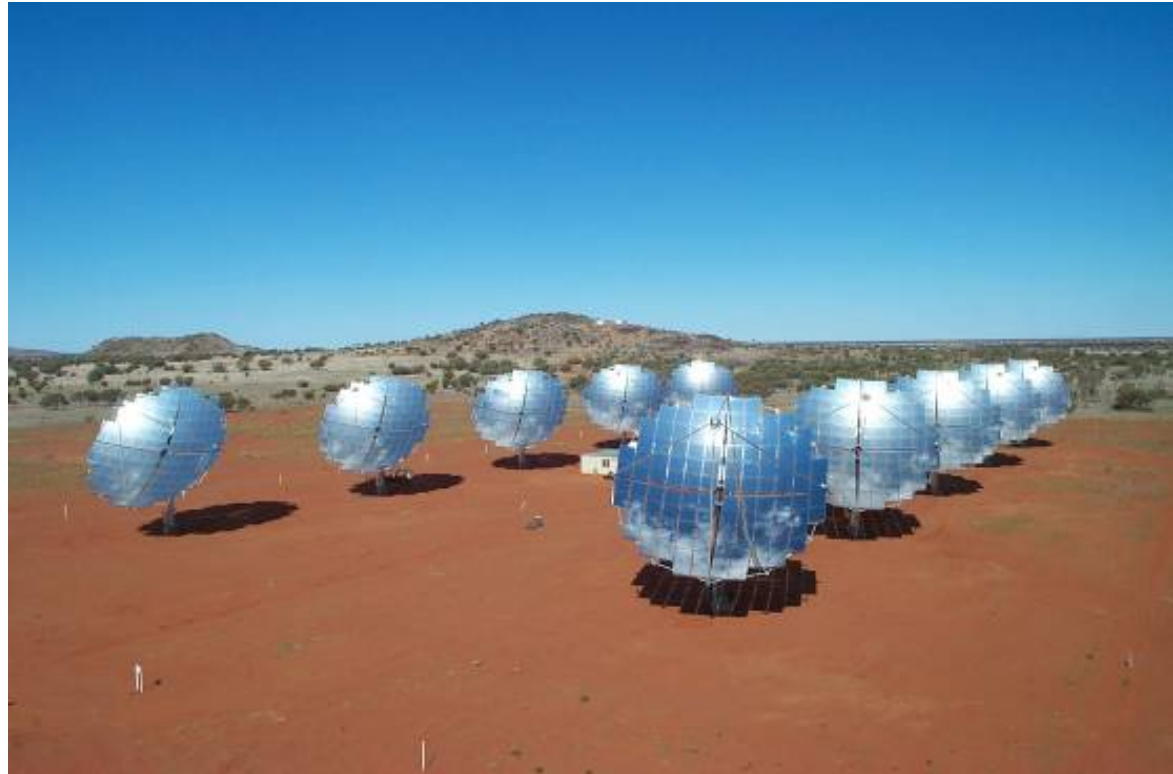
Solar Systems Pty Ltd: 220 kW PV Concentrator power plant at the Pitjantjara lands
