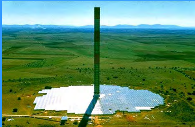
Manzanares 200 m high, 10 m diameter Collector 0.04 sq. km 50 kw, 130 J/kg, 1 Mg/s Spain 1982 to 1989
