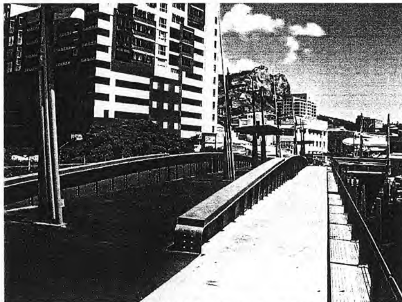
Photo 2 The refurbished deck looking west towards Castle Hill.
