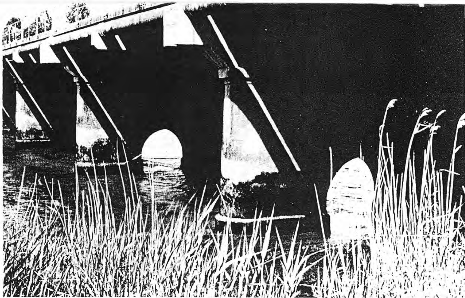
Fig. 133 Lamington Bridge, Maryborough, 1896, is one of the world's first concrete girder bridges.
