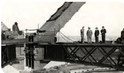
Engineers inspecting the Sydney Harbour Bridge
