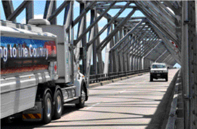
Traffic on the Burdekin River Bridge
