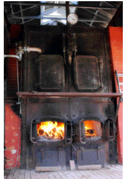
Millewa 'A' boiler in operation in September 2010 after re-tubing
