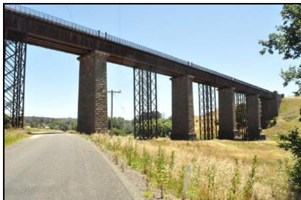
The Taradale Viaduct today. Its original wrought-iron continuous tubular beams were propped by intermediate piers built in 1933-1934.
