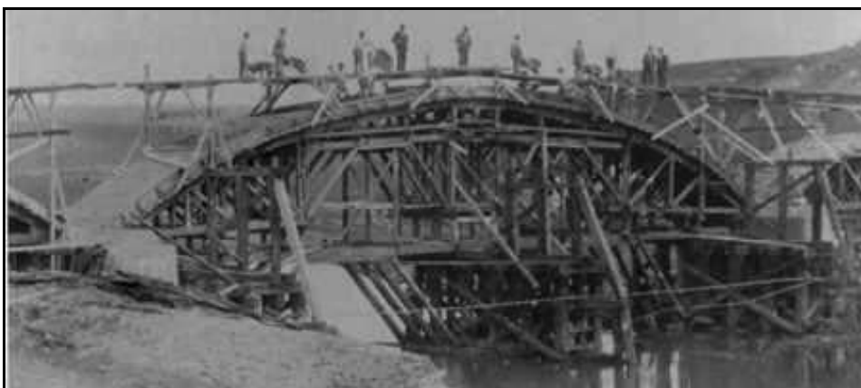
Placing concrete in the central span of the bridge, 1899.
