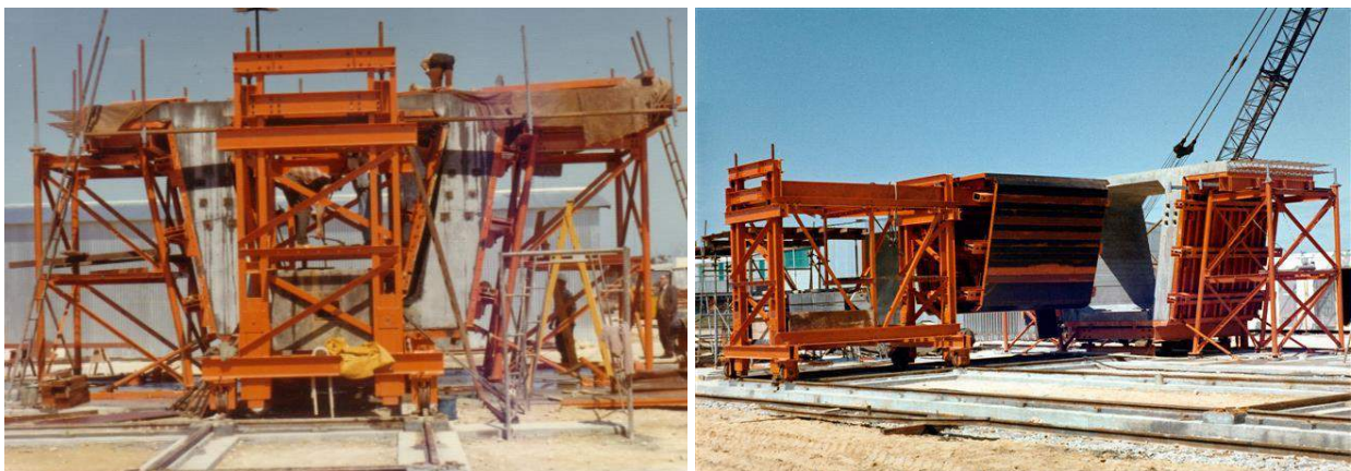
Figure 6. Precast beam unit travelling steel forms - internal form being released (Photos J O Clough & Son)
