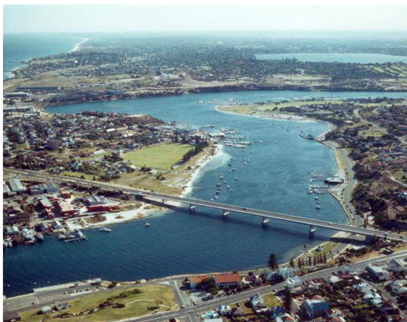
Figure 3. Aerial view of the Stirling Bridge looking north, on completion (Photo J O Clough & Son)
