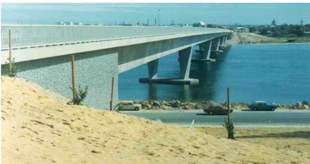
Figure 14. Completed bridge, 1974 (Photo courtesy J O Clough & Son)
