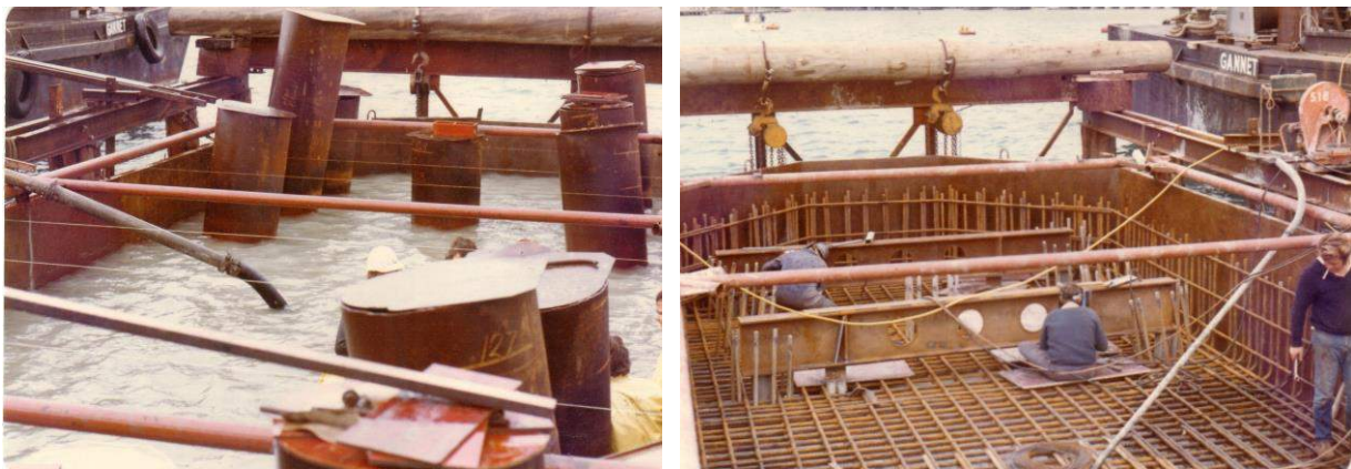
Figure 7. Left: Dewatering the pile cap; Right: Placing the hanger beams to transfer pile cap loads to the steel piles (Photos J O Clough & Son)
