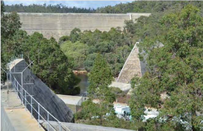
A central one-third section of the original Victoria Dam was blasted to create a channel for overflow water from the replacement dam 300 metres upstream.
