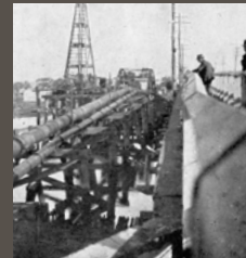
The original 12-inch main and subsequent 21-inch main pipelines from Victoria Reservoir cross the Swan River at the Causeway bridge.
