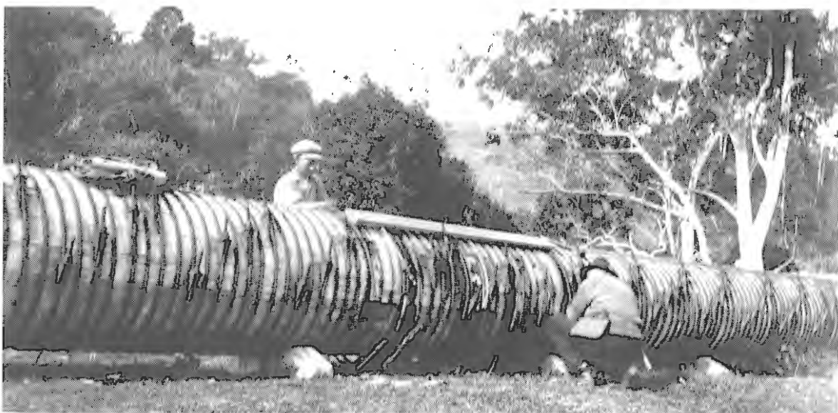
The original Chichester gravitation pipeline was made of wood staving between the Dam and Dungog. The pipe was paralleled with a steel pipe in the 1940s and subsequently abandoned.
