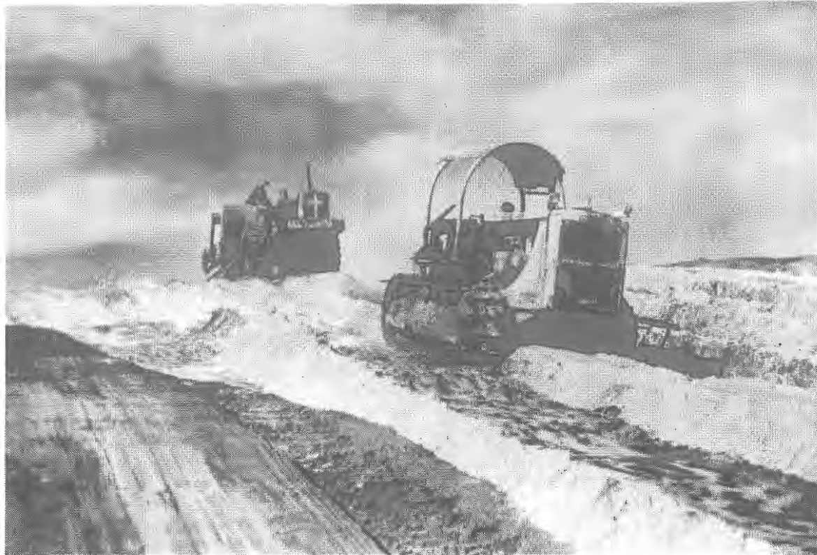
Dozer and scraper constructing the Grahamstown Embankment, 1959. HDW
