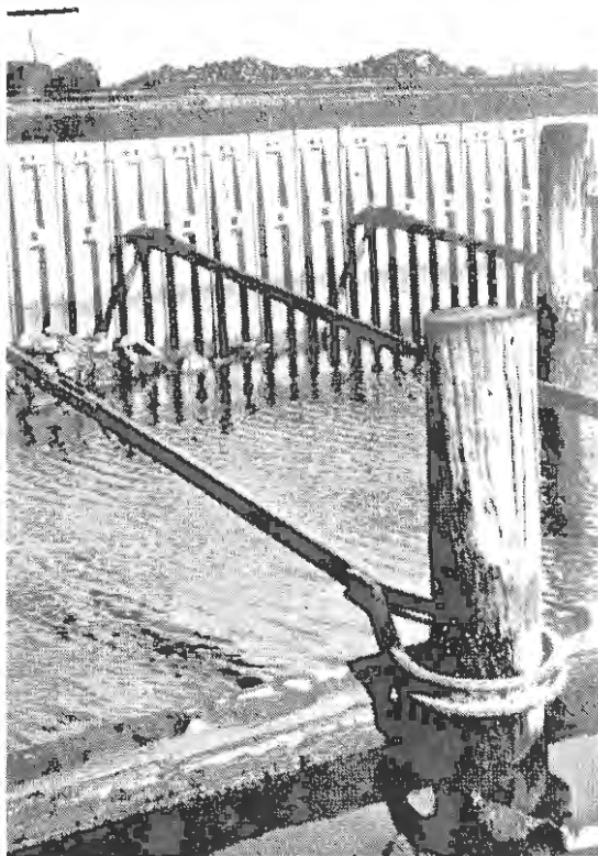
Wharf construction, West Basin, about 1915 — the pioneer use of reinforced precast concrete slabs.
