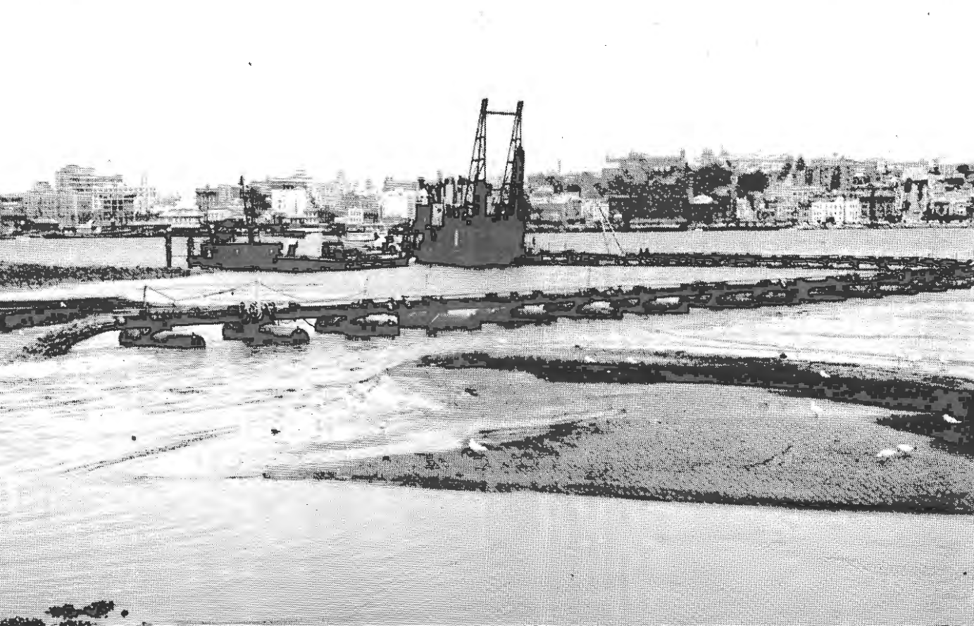
Cutter Suction Dredge I pumping fill at Stockton for the new passenger ferry jetty, 1957.
