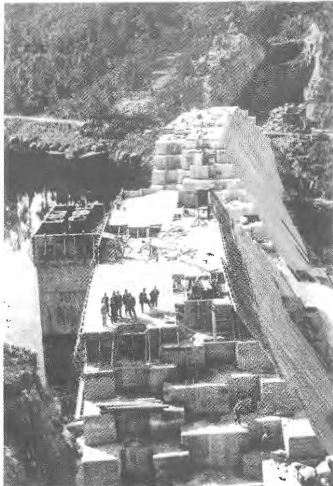
The concrete blocks which form the wall of Chichester Dam, 1924. HDW
