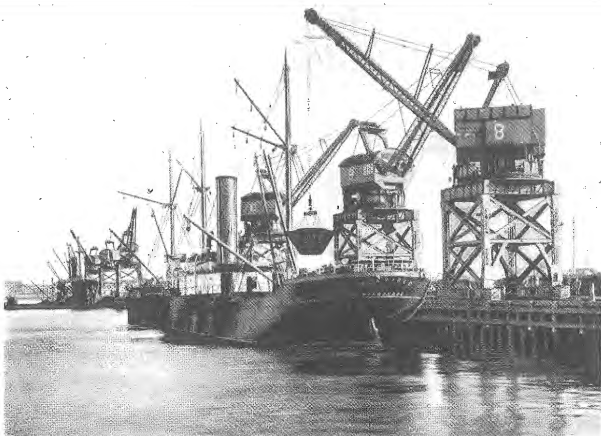
Fifteen-ton electric travelling cranes, Basin Wharf, west side, about 1915.
